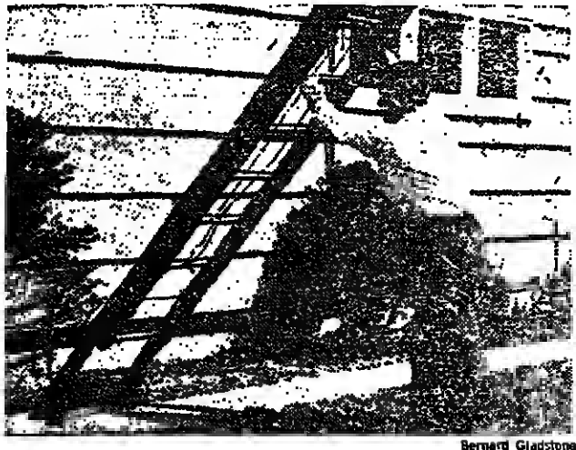
To raise a ladder to its vertical position butt bottom end against base of wall, then walk toward wall while moving hands from rung to rung.
